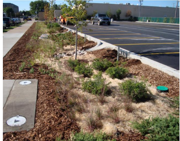
Bioretention Facility, UW-Stevens Point
