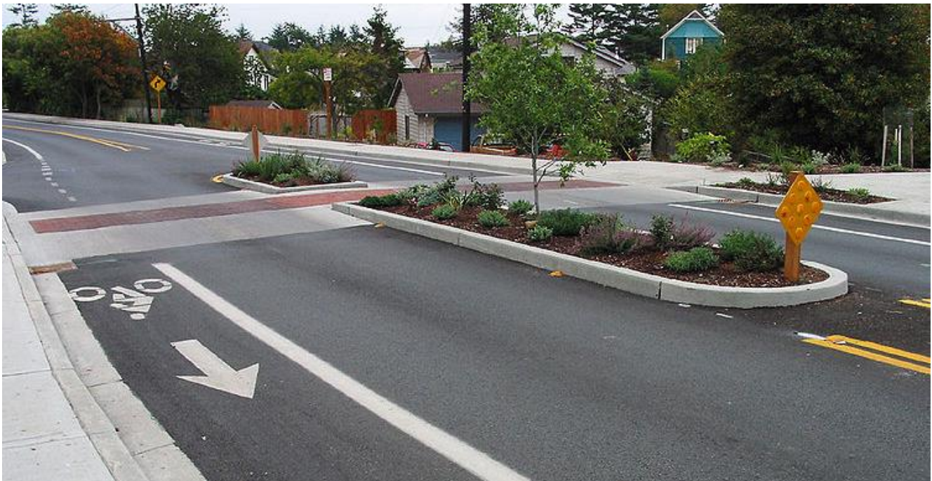
This mid-block crossing includes a raised crosswalk, colored pavement, landscaped refuge islands, and signage.
