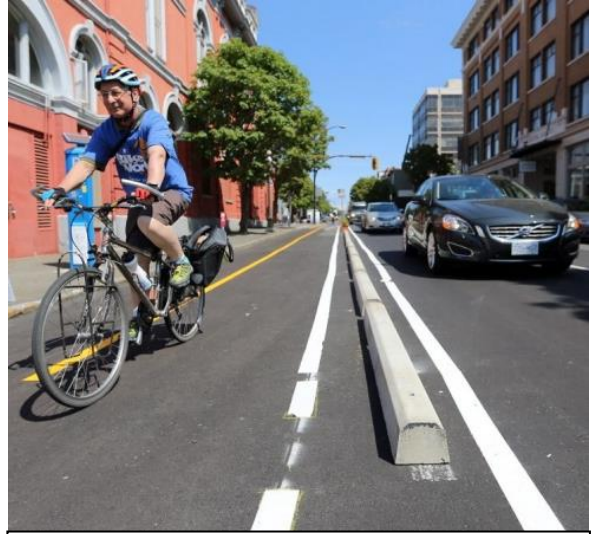
This separated bicycle lane in utilizes wheel stops and paint for a low-cost retrofit.
