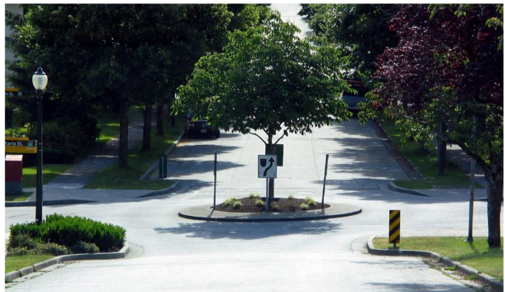
Traffic circles slow vehicles at unsignaled intersections.
