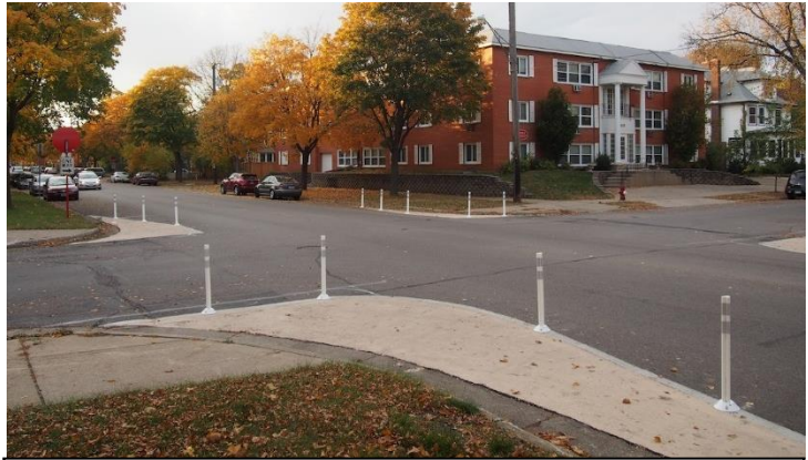
This curb extension in Minneapolis utilizes colored paint and candlestick posts as an inexpensive retrofit.
