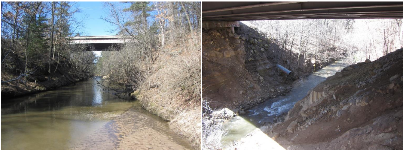
Above Left: View of Otter Creek looking north under HW12. Right: Constraints under HW12 bridge.
